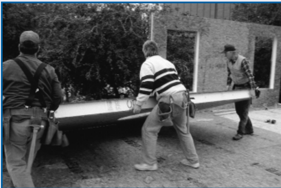
Figure 1. Fabricated SIP wall panels. (Photo courtesy of SIPA.)
