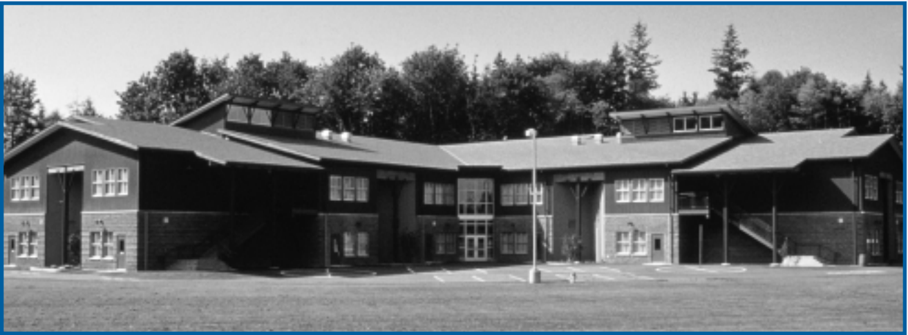
Figure 2. Pine Crest Elementary School, Bremerton, Wash., is an example of a nonresidential building constructed with SIPs. (Photo courtesy of SIPA.)
